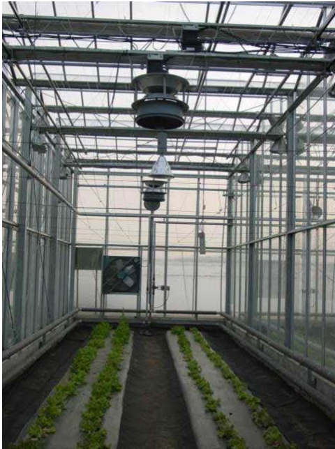
Fig. 1. Air mixing using air-circulation fan
